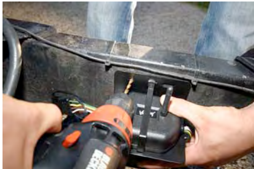
A high speed drill bit is used to drill holes that are slightly smaller than the mounting screws.
